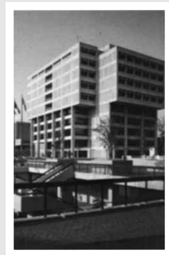
Civic Center Government Building, Baton Rouge, La.
