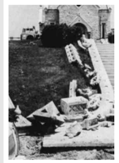
Before. Rails destroyed by a tornado.
