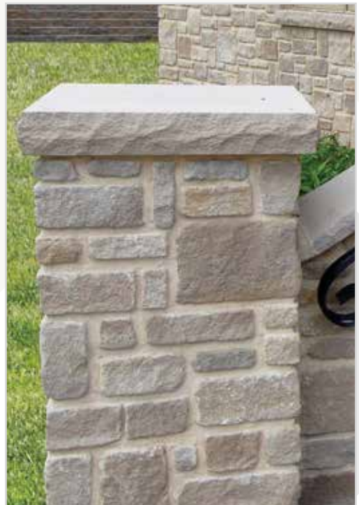
Rock face pier cap.
