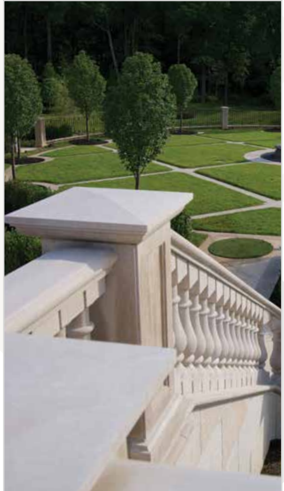
Custom pier caps and wall caps.
