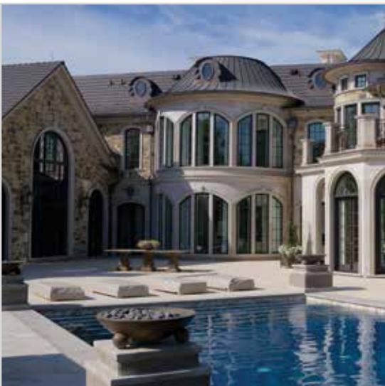
Custom pool coping and window trim.
