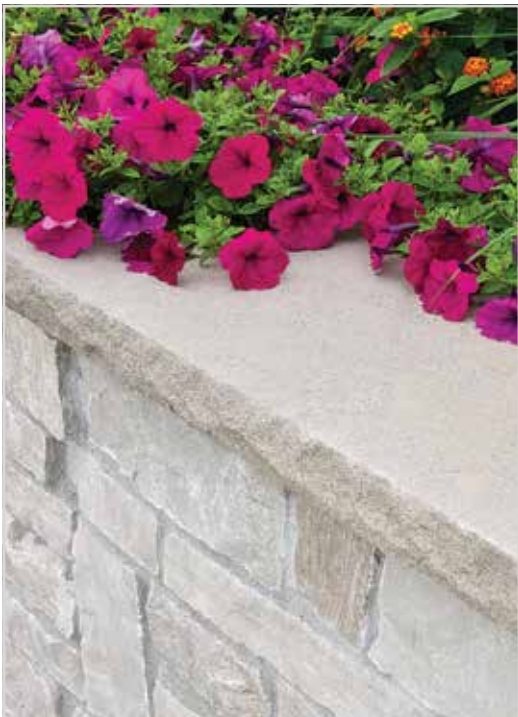
Rock face wall cap.
