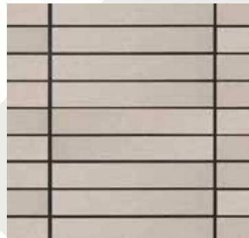
A pattern where the facing stone is laid with all joints aligned.
