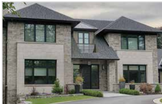
Vanderbilt veneer shown in running bond pattern to accent lower windows.
